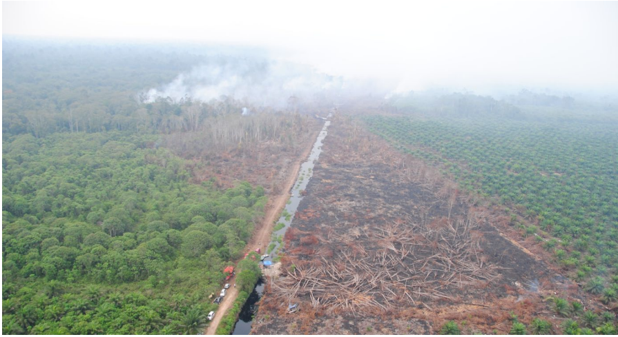
Figure 3-33a: Area of peat swamp forest degraded by fire along an abandoned logging canal in Raja Musa Forest Reserve, Malaysia in 2012
