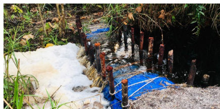
Figure 3-24: Sandbag block wrapped in tarpaulin sheet to prevent erosion when water flows over it
