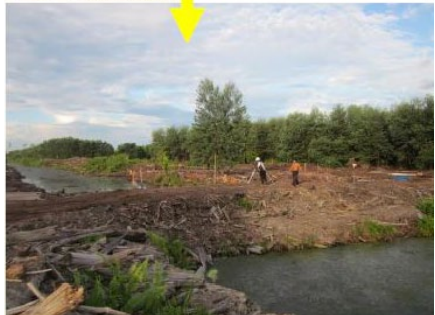
Figure 3-13: Large canal blocked by compacted peat block (Source: Wardhana, B., 2016)
