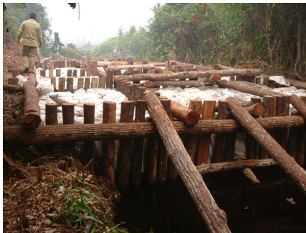
Figure 3-20: Plank Block in small drain. (Photo courtesy of Alue Dohong)
