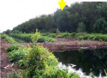
Figure 3-13: Large canal blocked by compacted peat block (Source: Wardhana, B., 2016)
