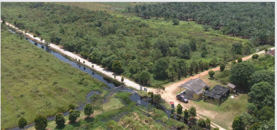
Figure 5-13c: RMFR rehabilitation site in 2018.
