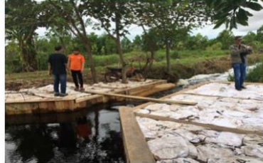
Figure 3-27: Block and Spillway design for medium block (Note: Relatively high level of spillway) (Source: BRG, 2018)
