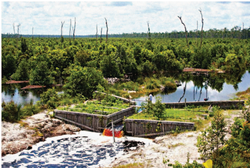
Figure 3-10: Dam constructed to block a former logging canal to restore peat swamp water levels.
