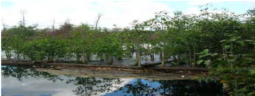
Figure 3-28: Sandbag block, topped by Geotextile and planted with trees (Source: Wardhana, B., 2016)
