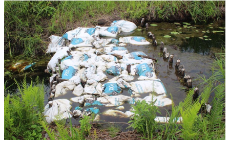
Figure 3-15: Sandbag block in large canal.
