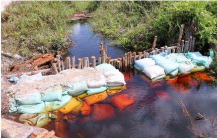
Figure 3-14: A medium-width ditch blocked with sandbags and wooden posts.
