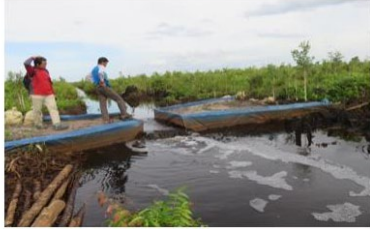
Figure 3-27: Block and Spillway design for medium block (Note: Relatively high level of spillway) (Source: BRG, 2018)
