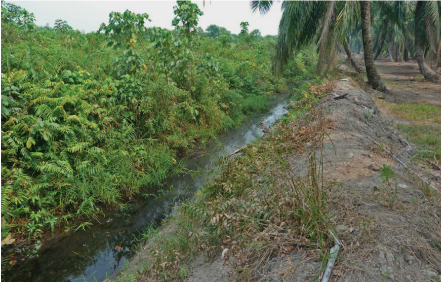
Figure 3-38a: Plantation perimeter drain in 2012 maintained with low water level led to drainage of adjacent peat swamp forest and was root cause of regular fires and poor forest growth.
