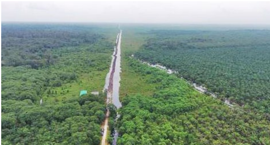
Figure 3-33b: Same area after construction of rockfill dam and natural regeneration over five years.
