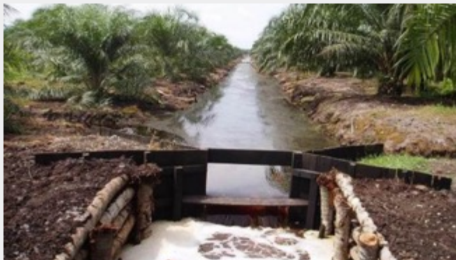
Figure 4: Water control structures (Credit: Left photo courtesy of Ministry of Environment and Forestry, Indonesia and right photo courtesy of United Plantation Berhad)
