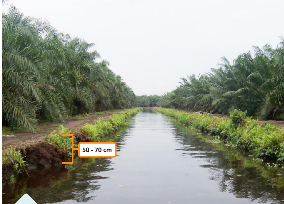
Figure 1: Water measured at collection drain needs to be in a range of 50 – 70 cm (Credit: Global Environment Centre, GEC)
